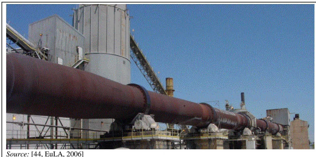
Figure 2.31: Example of a long rotary kiln used in lime manufacture
