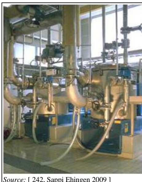
Figure 4.7: Pressure screens for final screening
