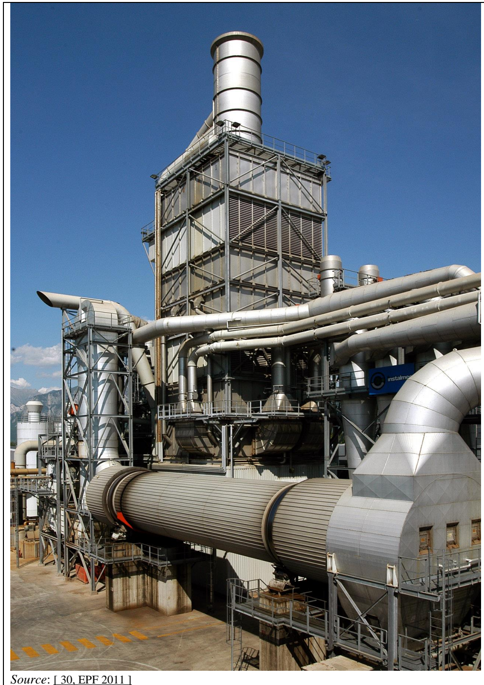
Figure 2.5: Rotary dryer
