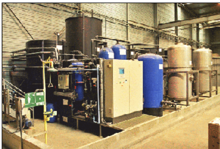
Figure 2.43: Example of waste water treatment plant using ion exchange (Productmetal S.A. and Agence de l'eau Seine-Normandie)
