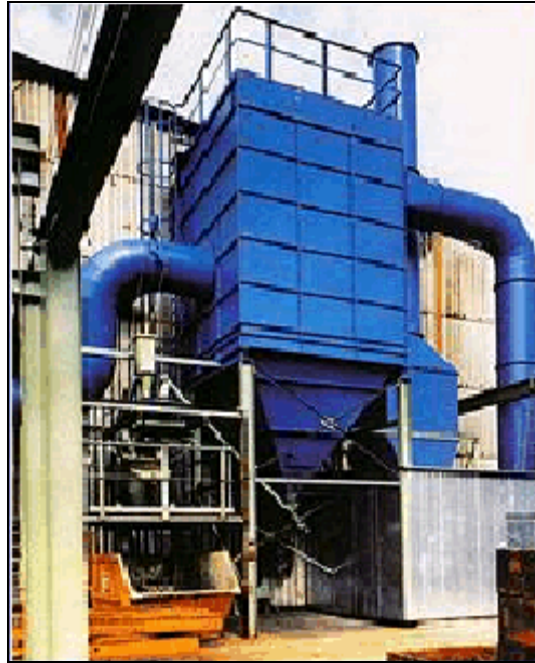
Figure 4.28: Picture of an industrial baghouse
