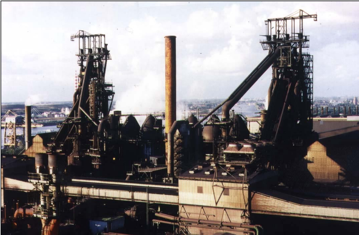
Figure 7.1 : : General view of two blast furnaces with three hot stoves each and the stack for the waste gas from the hot stoves
