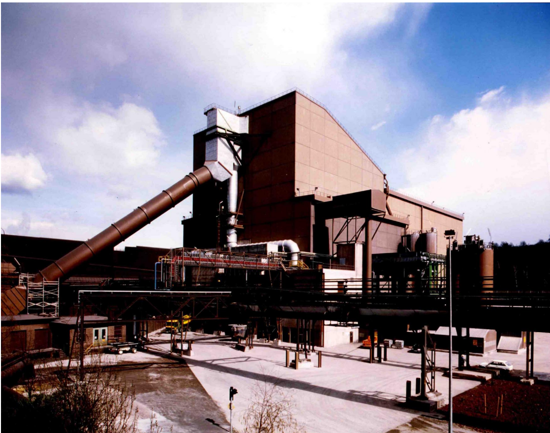
Figure 9.1 : Electric arc furnace plant
