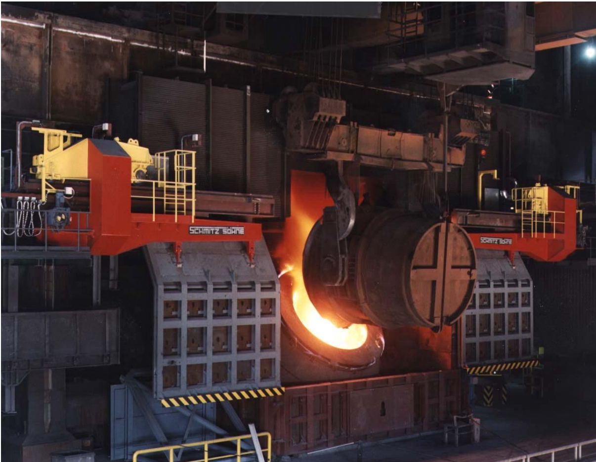
Figure 8.1 : Basic oxygen furnace at the moment of charging hot metal
