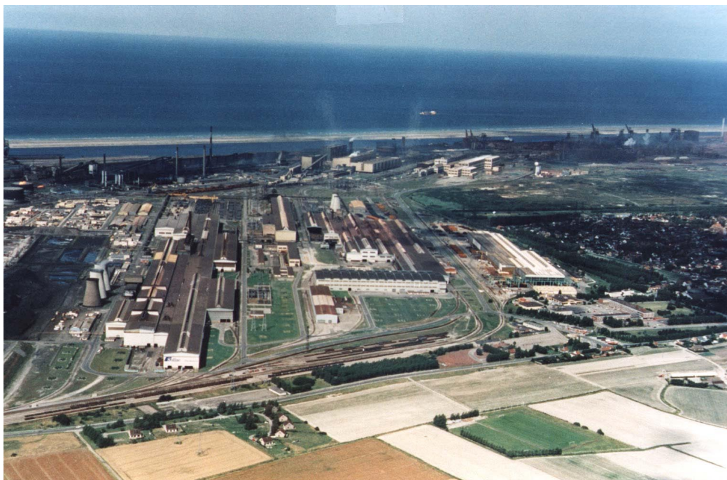
Figure 3.2 : Aerial view of an integrated steelworks located near the coast
