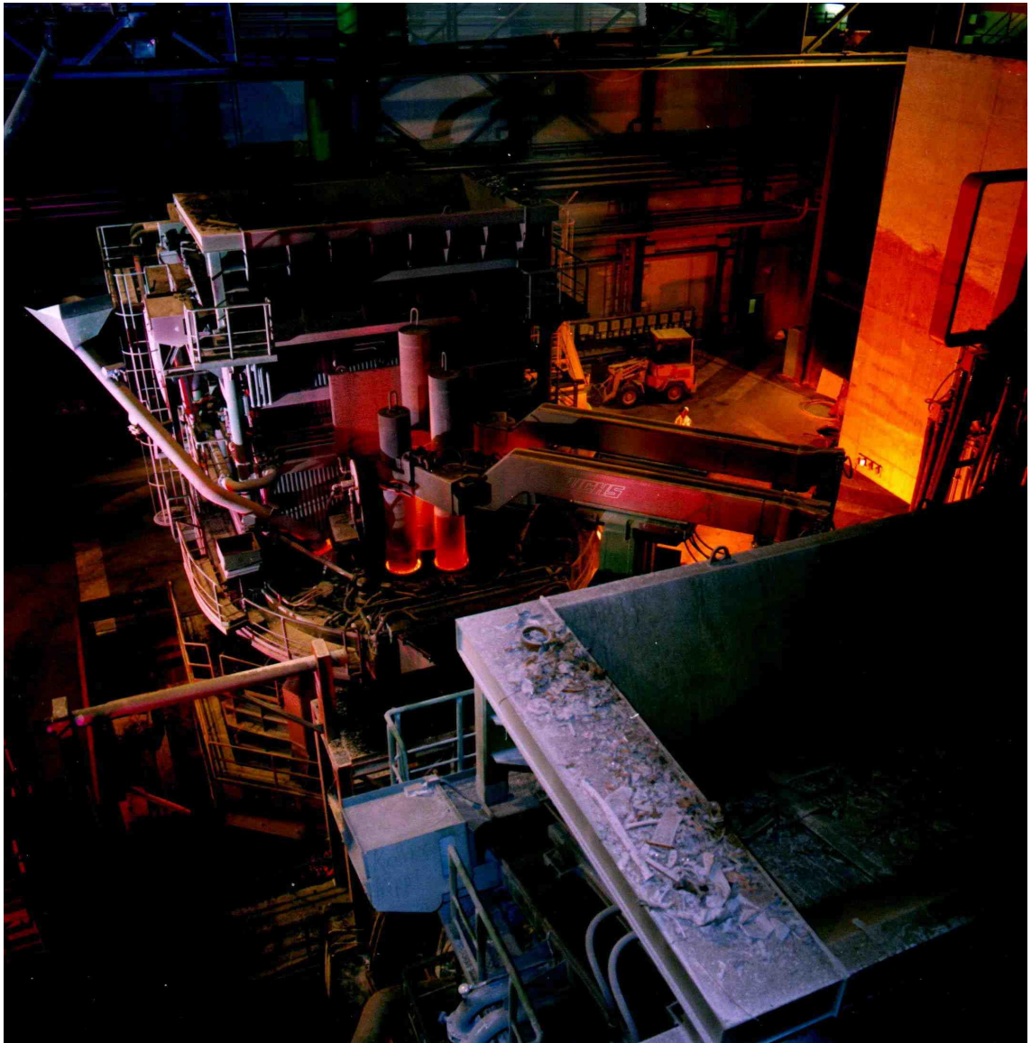
Figure 9.2 : Electric arc furnace with three electrodes and (in the foreground) a shaft for scrap charging
