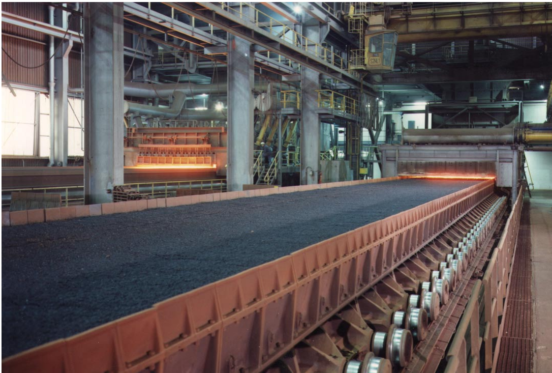
Figure 4.1 : Photograph of a sinter strand with the charging facility (drums or chutes) and the ignition canopy at the starting end
