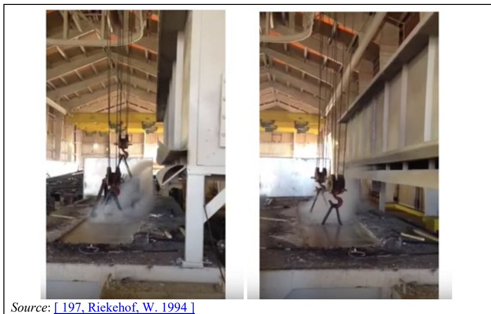
Figure 8.50: Lip extraction at a batch galvanising plant
