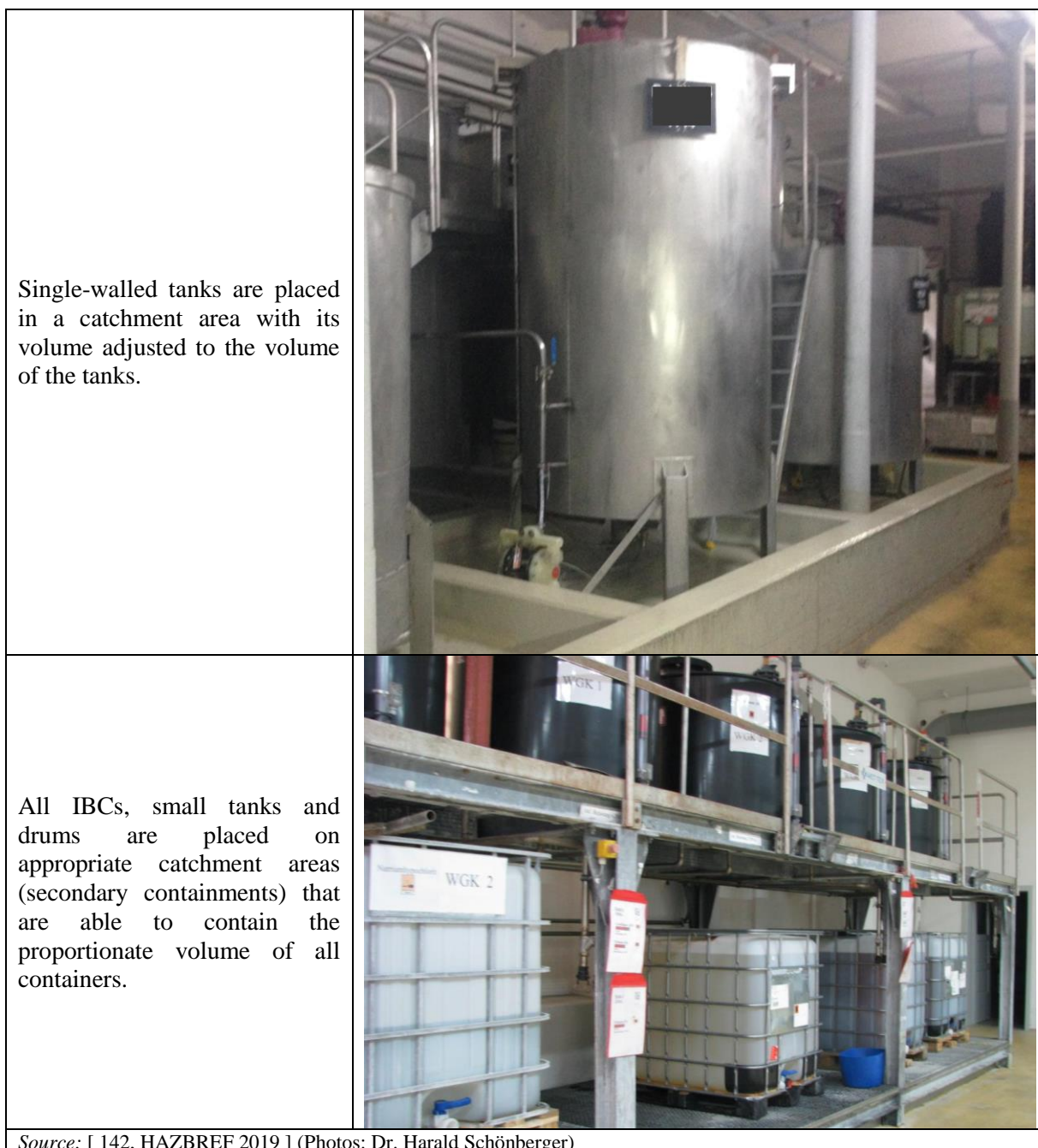
Figure 4.13: Measures for proper storage and handling of chemical products
