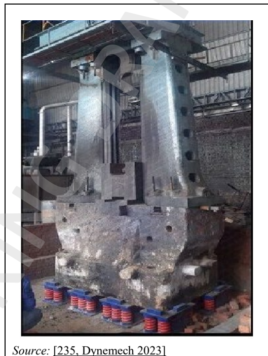
Figure 3.68: Closed-die hammer (3.5 tonne) on spring viscous isolators
