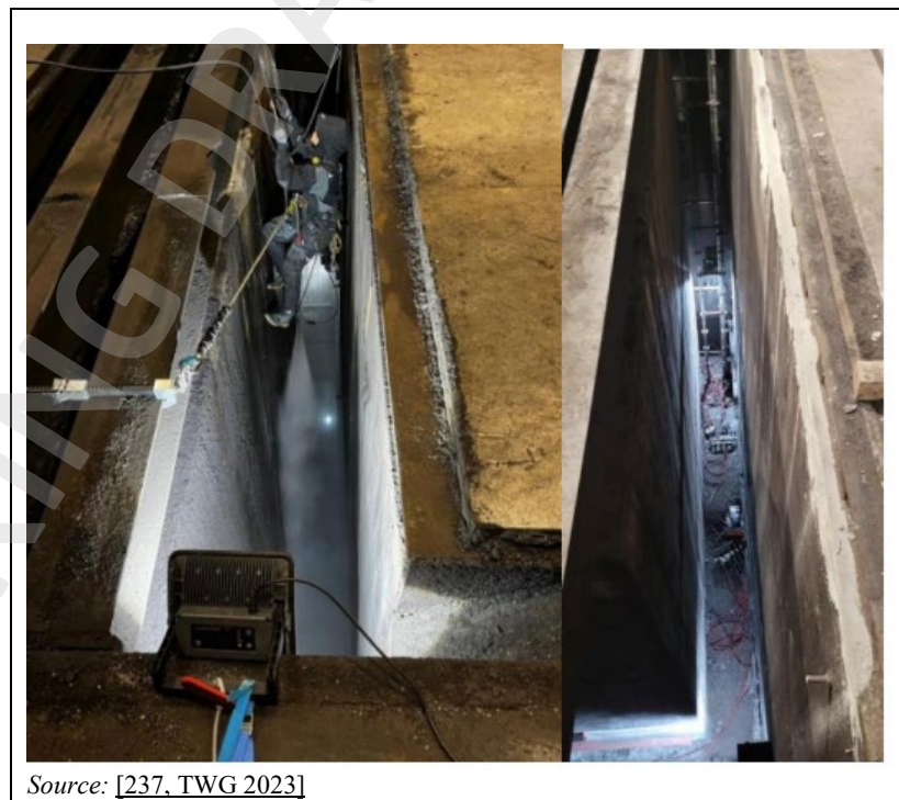
Figure 3.70: Foundation of a 6-tonne hammer at Plant DE002
