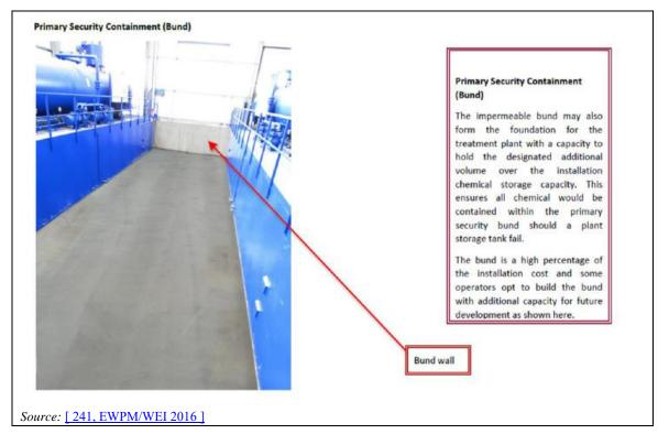
Figure 15.21: Design examples for process containment
