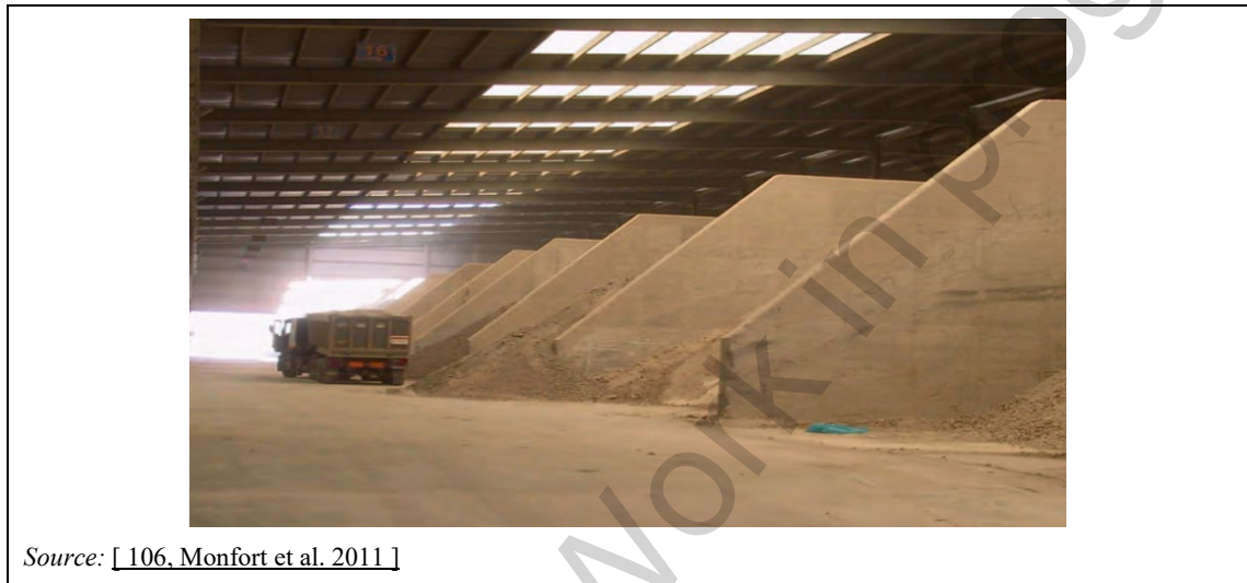
Figure 2-35: Raw material storage
