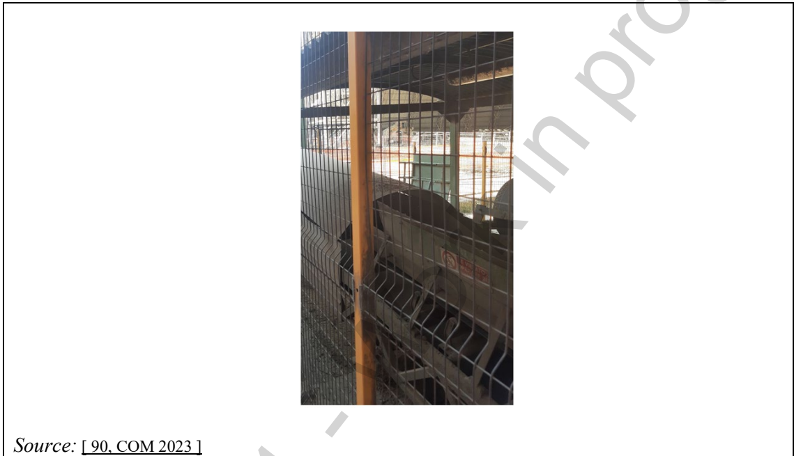
Figure 4-14: Covered conveyor belt
