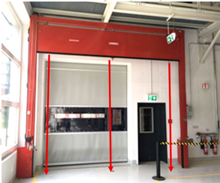
Figure 4-3: Bulkhead for sectional door and pass door
